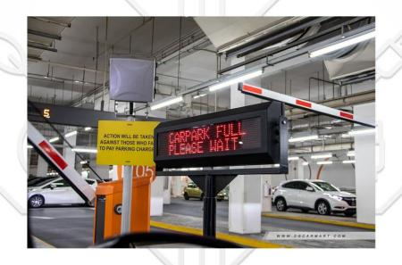
Equipping public parking lots with intelligent management and guidance systems can reduce parking space problems. By using parking automation, not only the running costs are reduced, but it can also save the visitors' time. The use of new technologies such as image processing and the use of sensors that exist in the place, determines how many empty spaces there are. Also, this system can be used in security cases.
